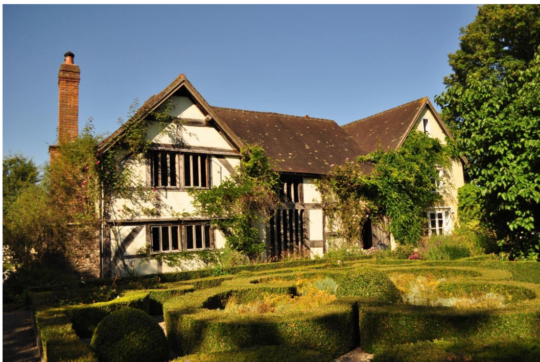
Figure 5. The Marsh, Eyton, Herefordshire. South elevation of the 15 th century late medieval open hall house. The earlier crosswing is on the left. The crosswing on the right, which stands on the site of the lost service wing, is a modern construction.
