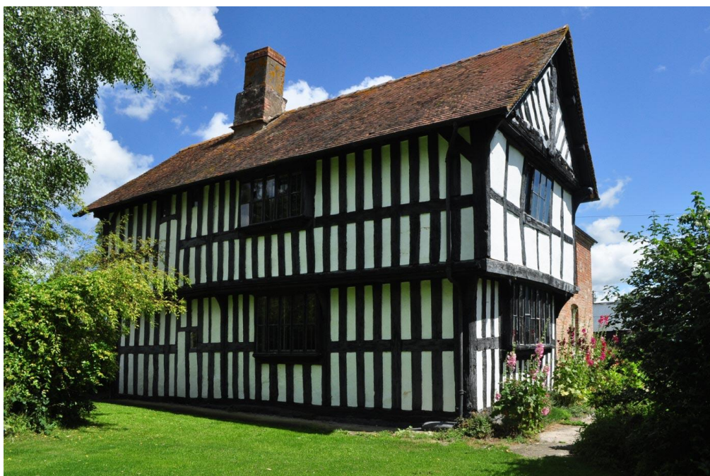
Figure 8. Eyton Court, Eyton, Herefordshire. The surviving crosswing of the early 16 th century house built by Thomas Hakluyt. The close studding continues around the back of the wing.
