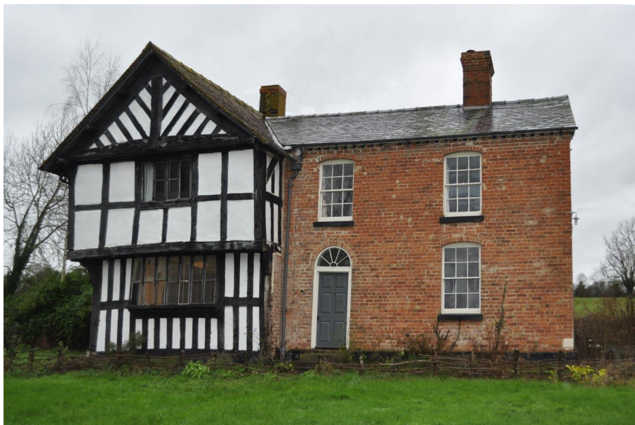
Figure 1. Eyton Court, Eyton, Herefordshire. South elevation showing the later brick range abutting the side of the timber-framed crosswing. The original close-studding and oriel window at first-floor level have been replaced with large-panel framing, probably in the 17th century.
