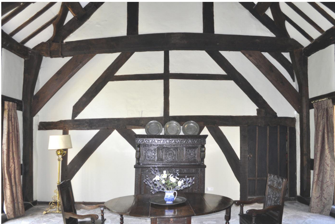
Figure 7. The Marsh, Eyton, Herefordshire. The interior of the open hall looking west to show the sidewall of the earlier crosswing with its embedded truss that formerly supported the roof of an earlier hall with a lower roof level.
