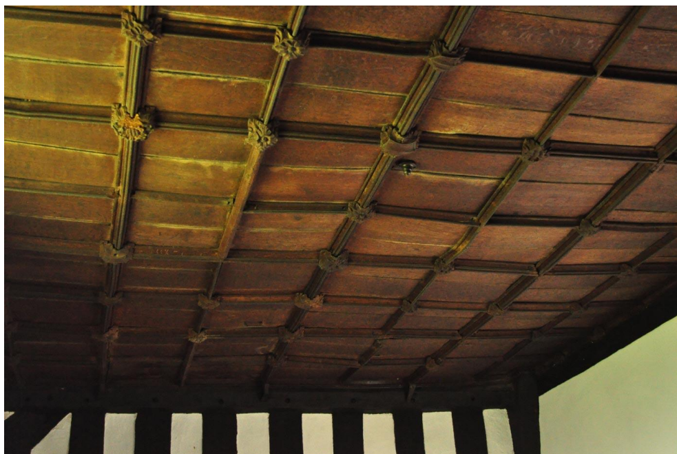
Figure 14. Eyton Court, Eyton, Herefordshire. Part of the first-floor panelled ceiling showing some of the surviving carved bosses.
