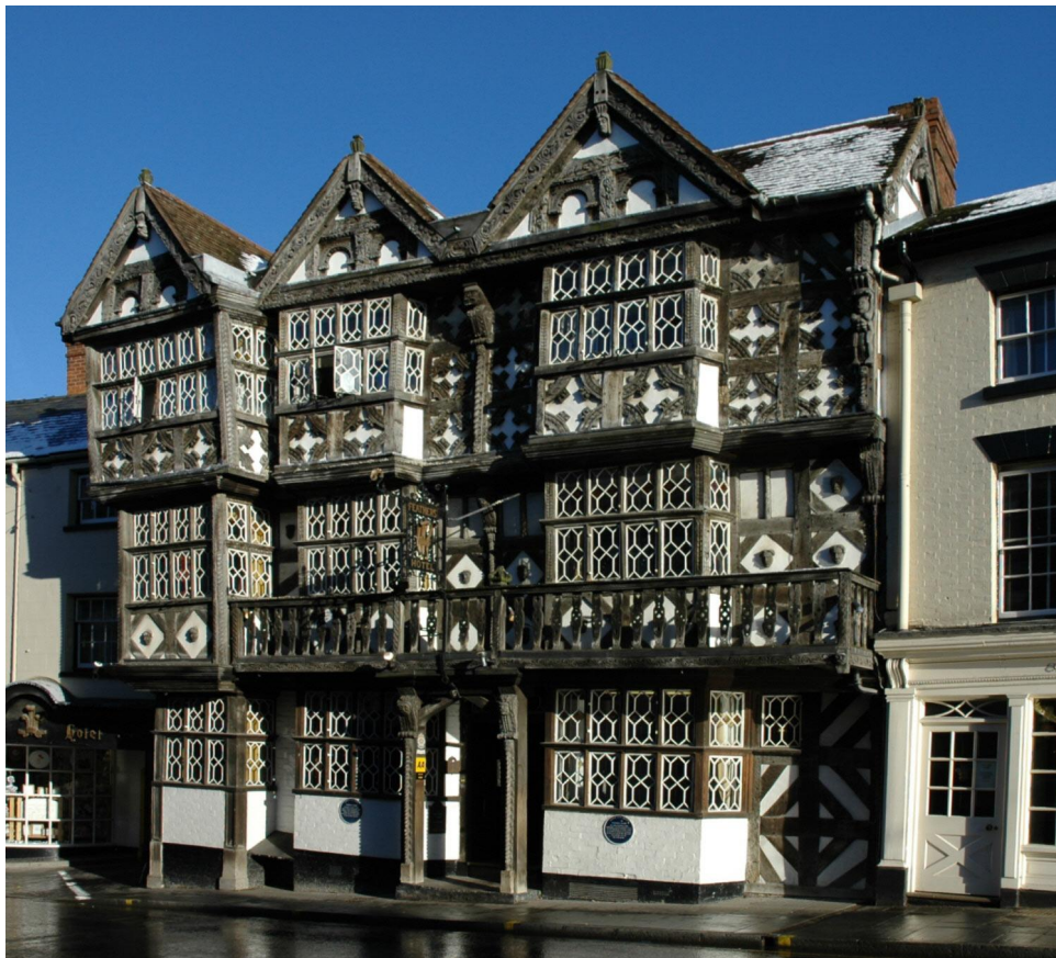
Figure 3. The Feathers Hotel, Ludlow, Shropshire. Behind the rich embellishment of the 17 th century façade lies the earlier, two-storey timber-framed town house of Thomas Hakluyt, Clerk to the Council of the Marches in Wales.
