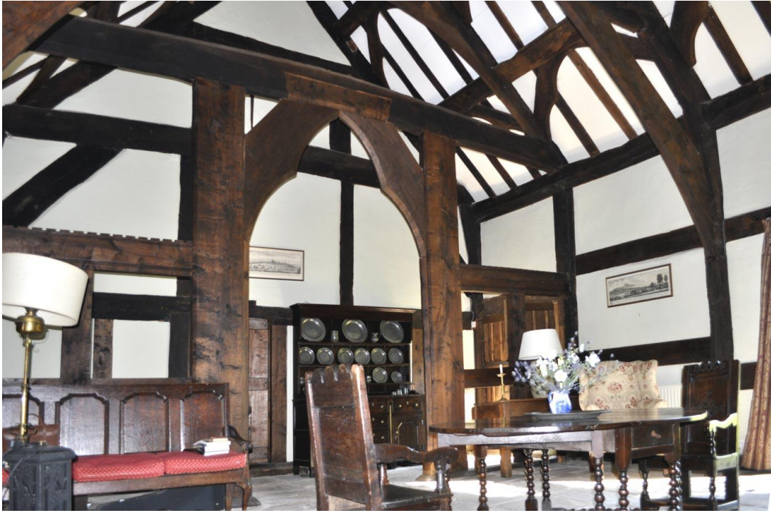
Figure 6. The Marsh, Eyton, Herefordshire. Interior view of the open hall looking east towards the reconstructed spere truss that separates the hall from the crosspassage.
