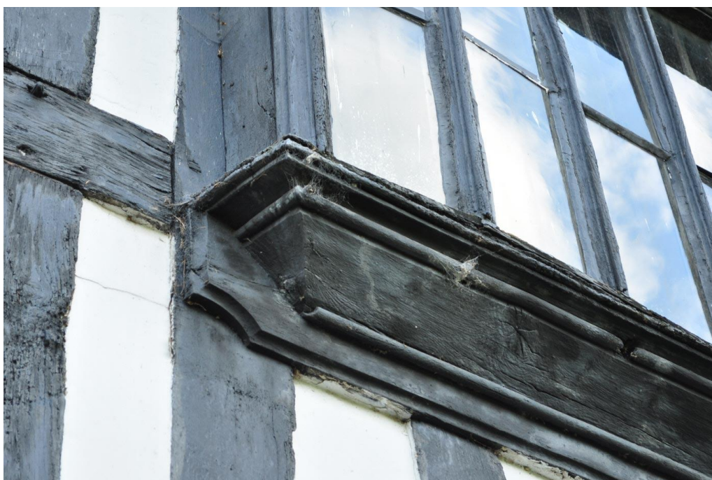
Figure 9. Eyton Court, Eyton, Herefordshire. The richly moulded sill on one of the five oriel windows.
